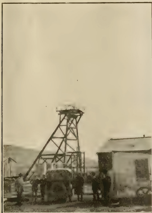
NO. 1. SHAFT HEADGEAR, EDEDALE.
